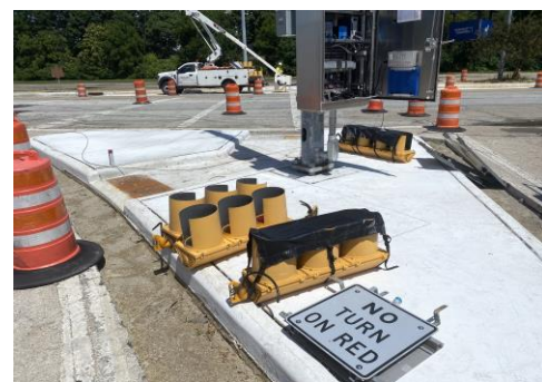
A view from the street of the construction
